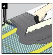
**Laying the tiles**Use a flexible tile adhesive to fix tiles straight over the heating
